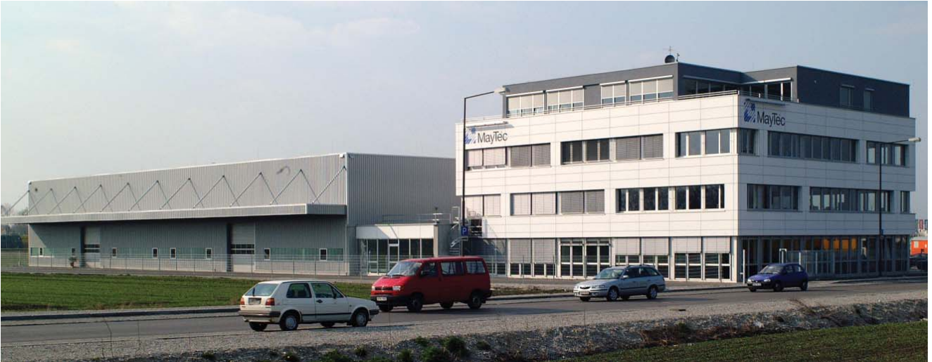
MayTec GmbH plant in Dachau
